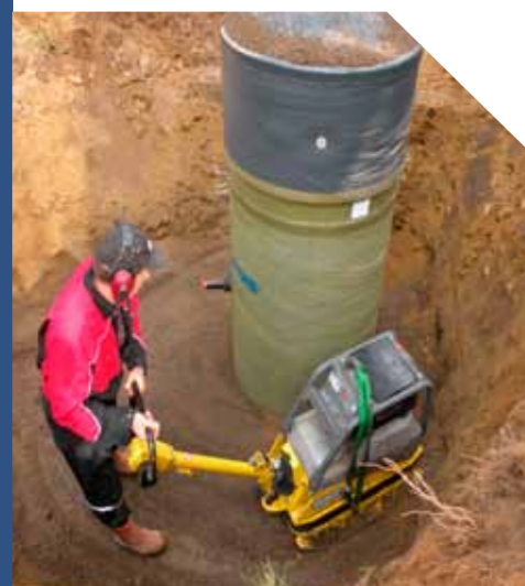
The pumping station tank requires a minimum of effort for installation.
